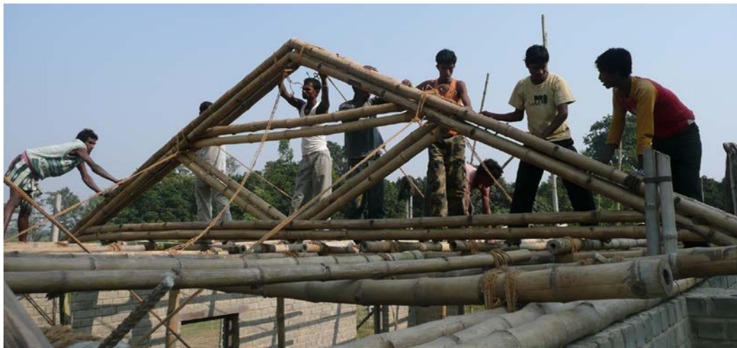
Figure 6. Bamboo truss being put on bamboo post (Author 2008)
