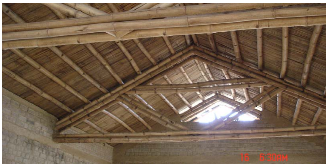
Figure 7. Bamboo roof on earth wall (Author 2008)
