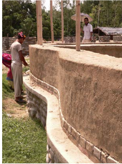
Figure 5. Bamboo reinforcement on walls (Author, 2008)
